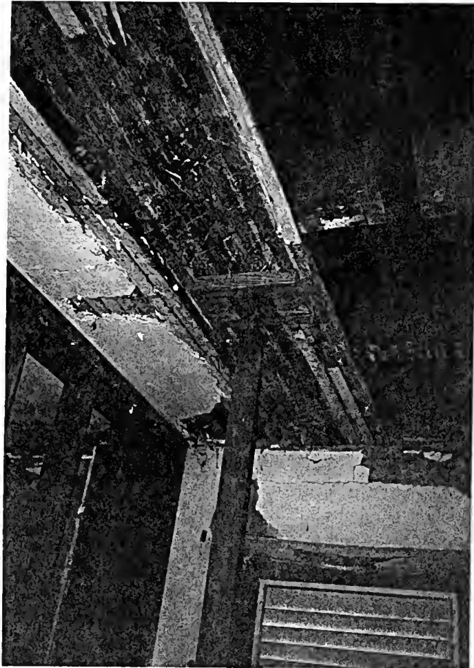
Figure 15: Second story summer beam with steel column as temporary additional support
